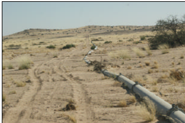
Plate 2.4: Southern wash section showing evidence of previous floods
