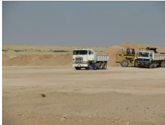
FIGURE 5.3 – BORROW PIT ON CURRENT ACCESS ROAD
