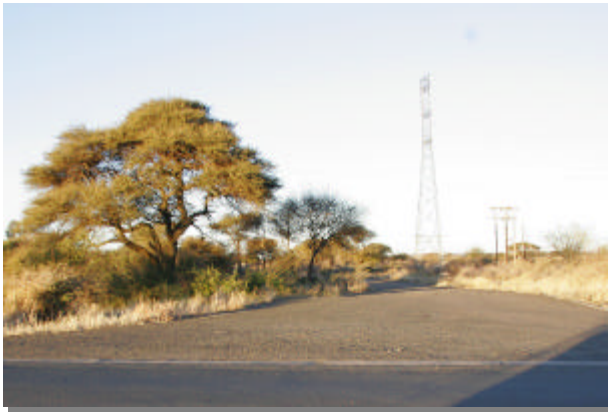
Photo 2: Power lines on the site.
