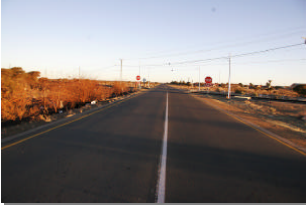
Photo 1: At-grade railway crossing on Roodepan Road
